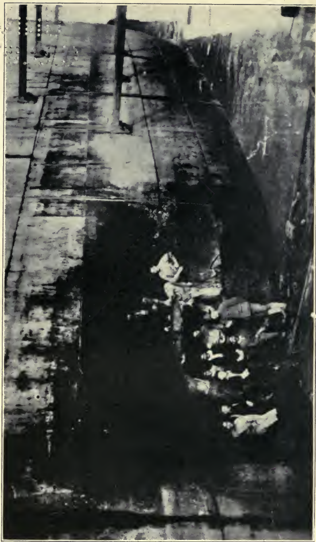
The Mount Vernon in dry-dock, showing the hole torn in her side by a torpedo
